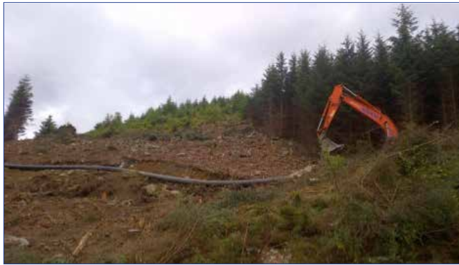
Laying the pipe down the hill.
