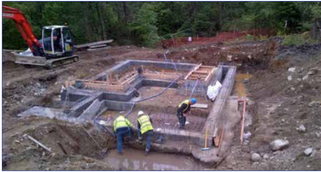
Building our turbine house - getting started.....
